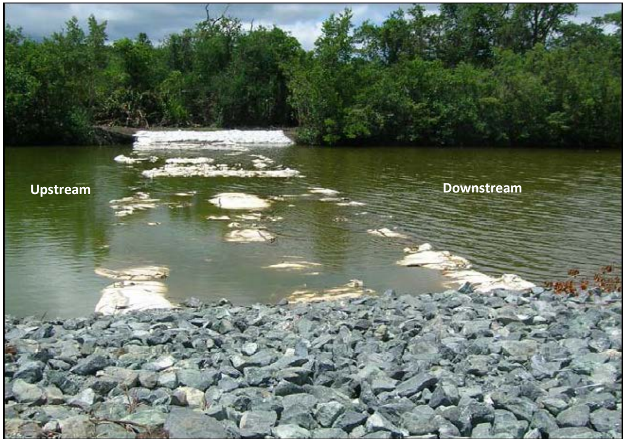
Figure 7. SWIM installed across the diversion channel (March 2007)
